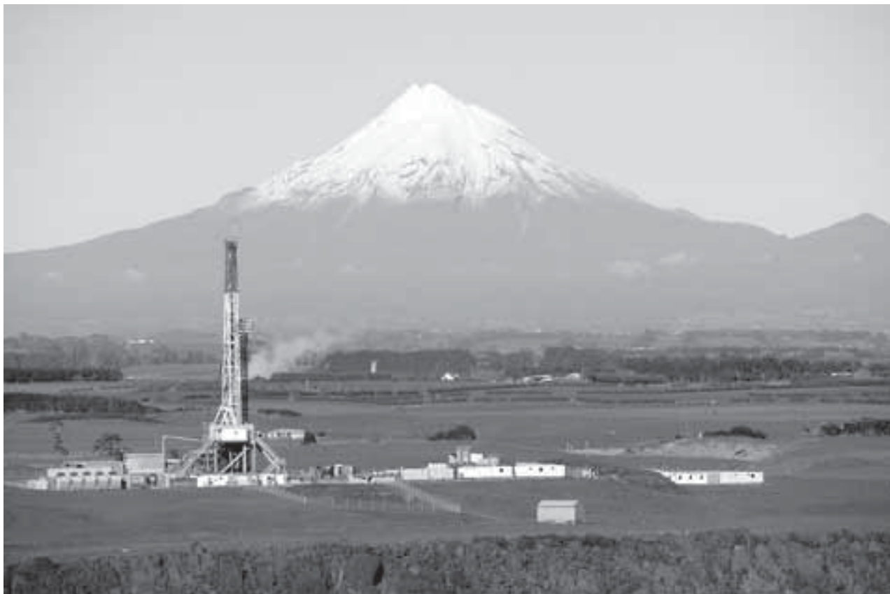
A drilling rig leased to Shell Todd Oil Services drilling for gas in the early stages of the Pohokura oil and gas field development at Motunui, north Taranaki, July 2007
