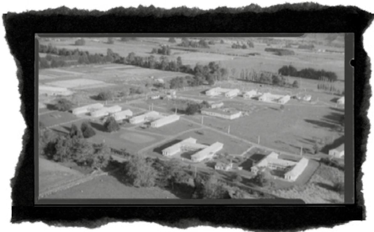
An aerial view of what was then called the Levin Hospital and Training School taken in the 1960s showing large ‘H’ shaped accommodation blocks on a large rural property.
